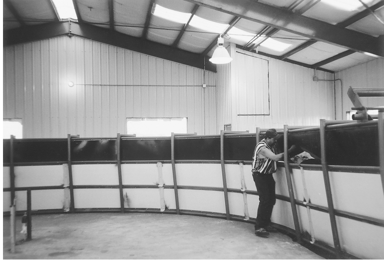
Figure 8.3. Cattle handling facility with white translucent plastic skylights to provide bright, shadow-free light. Solid sides on the single-file chute keep cattle calmer. To move the animals, the handler lifts up the rubber curtain along the top of the chute.
