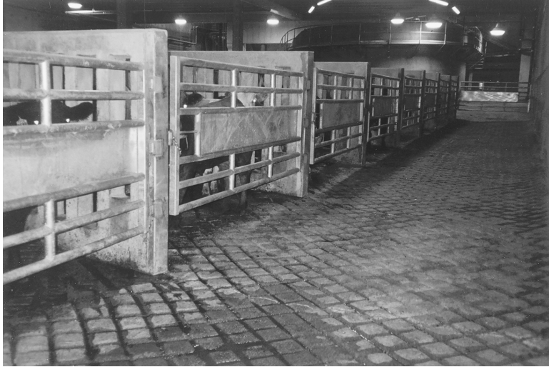
Figure 8.10. Nonslip flooring for beef cattle. This flooring is suitable for use in working, sorting, and loading areas. In places where cattle walk every day, such as dairies, smaller grooves should be used to prevent hoof damage.
